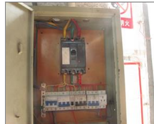
Photo of the inside of the main production hall IMG_9916.JPG
