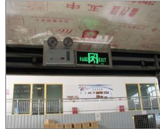
Photo of the inside of the main production hall IMG_9960.JPG
