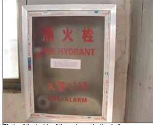
Photo of the inside of the main production hall IMG_9913.JPG
